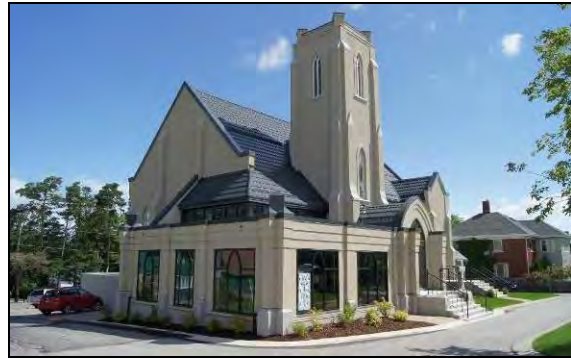
Retrofit – EIFS Simulated Stone
