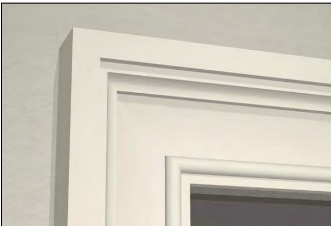
Figure 31: Trim - Typically flatter and narrower than headers or sills and used between the header and sill to improve the appearance of the jamb of a door or window. In some cases, trim may be used around the entire perimeter of a window. The term, "trim", may also be used instead of the term, "band". The framing or edging of openings are also known as casing.
