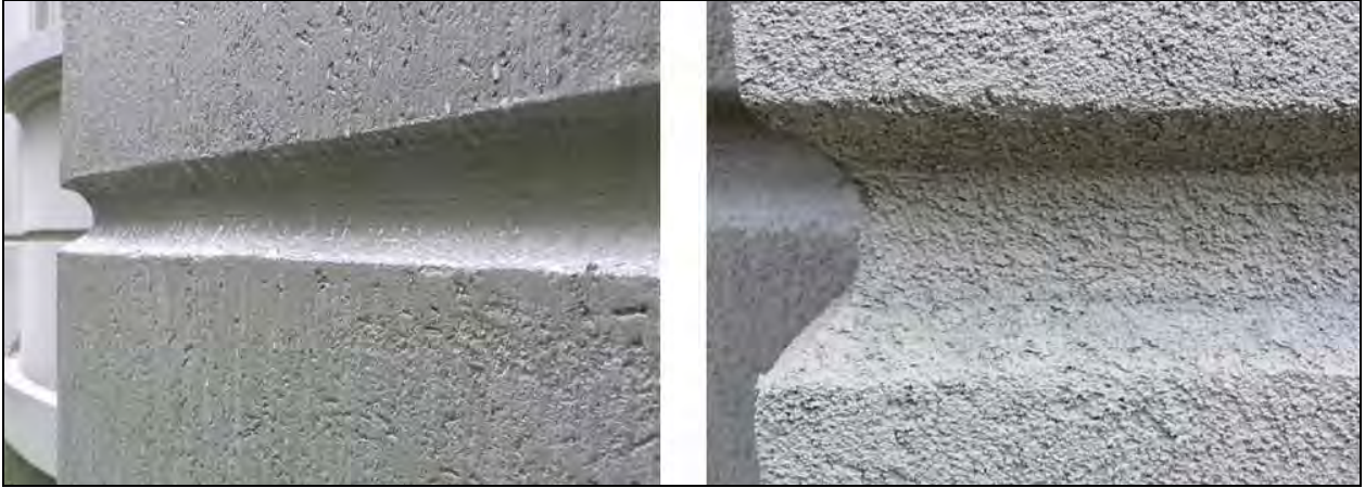
Figure 12: Ideal aesthetic reveal profiles (Left: Semi Rounded, Right: Trapezoid).
