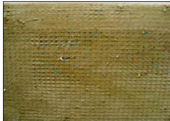
Inadequate Base Coat Coverage
