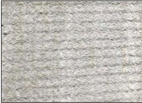
Acceptable Base Coat Coverage
